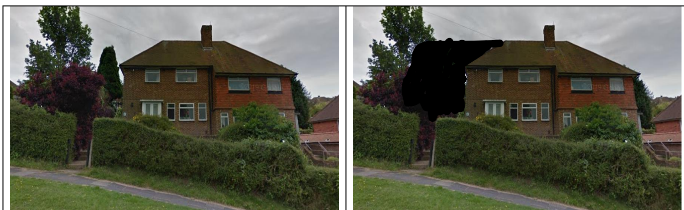
Fig. 6: view of Keymer Road from pavement level (before and after).
