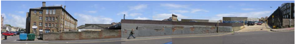
Southern Elevation – Kingswood Street, North
