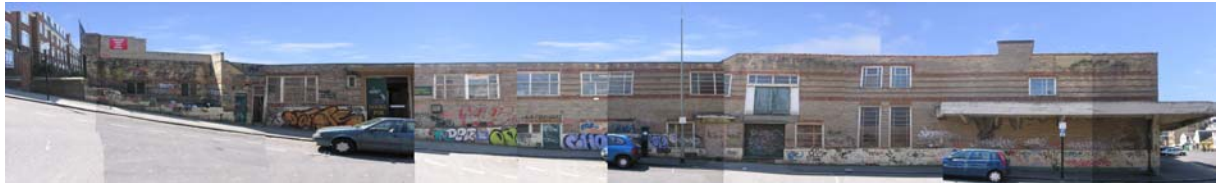
Northern Elevation – Morley Street, South
